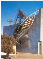
3520 Hayden Avenue, under construction
